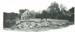
Material piled on building site—foundation in—November 3rd, 3 P. M.
