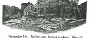
November 7th. Rafters and dormer in place. Most of roof sheathed.
